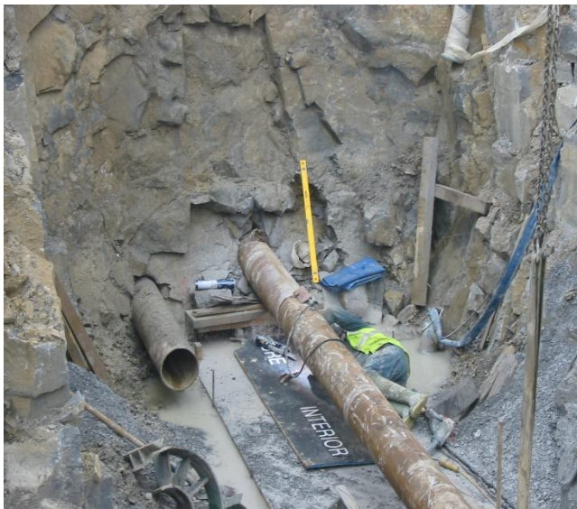
Welding of joint on surface water pipeline
