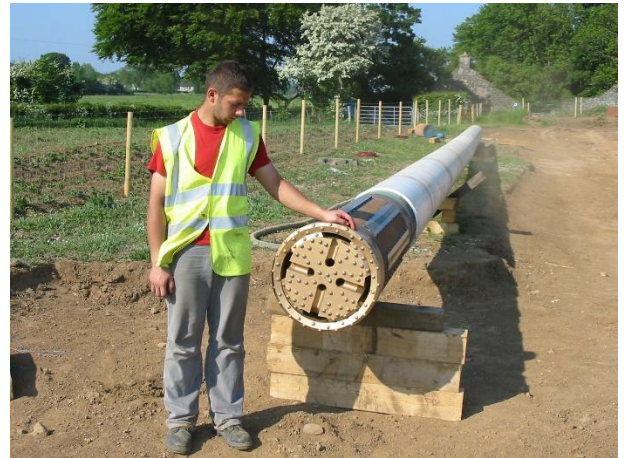
New rock head ready to install 457mm gas main
