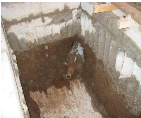
View of lead auger arriving in exit shaft
