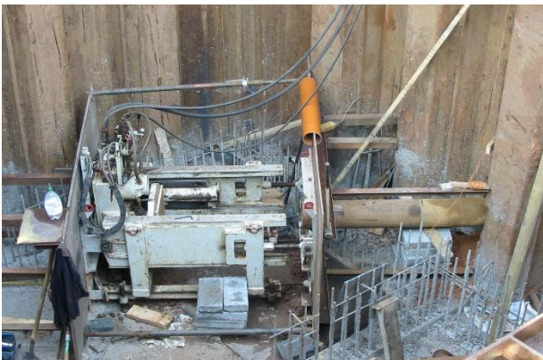
BM 400 set up in temporary works
