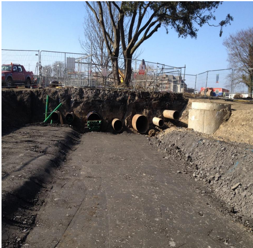
Pipes installed at Grangegorman, Dublin for service ducts.
