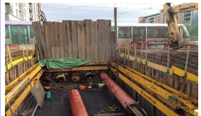
Luas crossings for service ducts at Mayor Street, Dublin.
