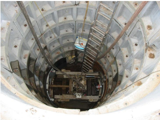
BM400 Set up in launch shaft
