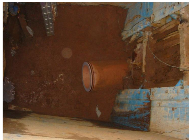
Pipe installed in exit shaft to line and level
